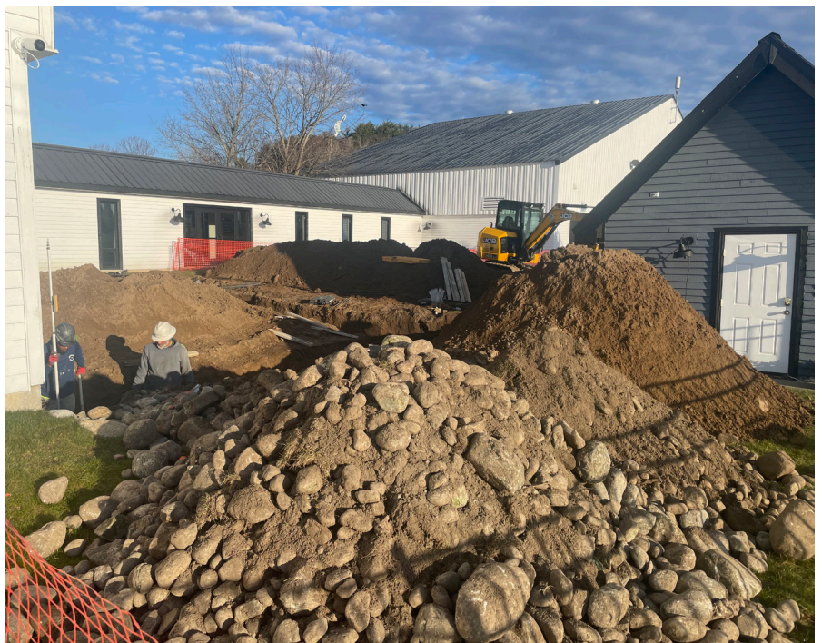
Construction has started this week on our new gymnasium
